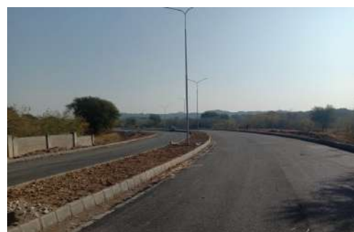
Roads Construction - Campus II
