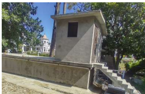
Reconstruction of Under Ground Water - Campus I
